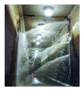
The condition of the internal galleries at John Day Dam raised immediate concerns for worker safety during the repairs.
